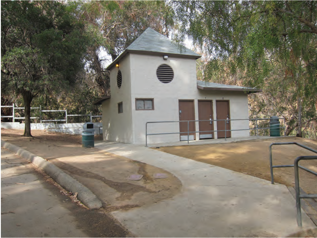
Existing onsite restroom facilities
