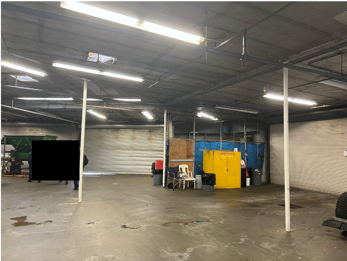
Image 11- Condition at Ground level storage
