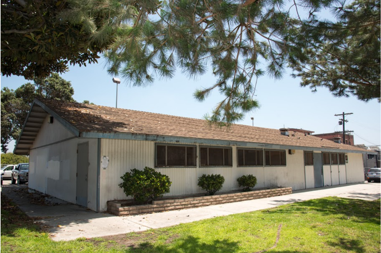
West face of the Center along Pacific Avenue
