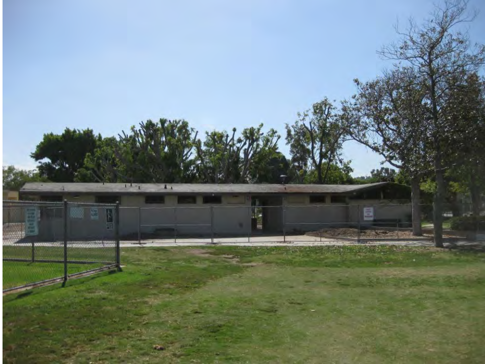
Plate 9. Restroom Facility, north side, view facing south
