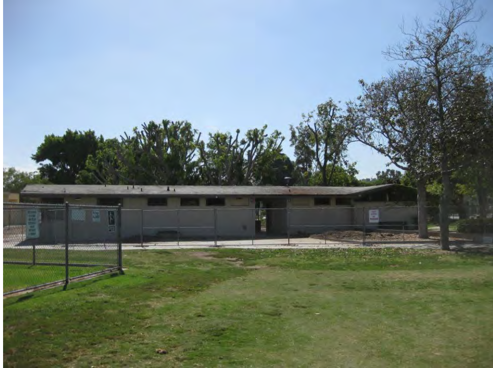
Plate 9. Restroom Facility, north side, view facing south
