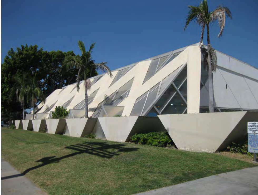
Plate 6. Celes King III Indoor Pool, south side, view facing northwest
