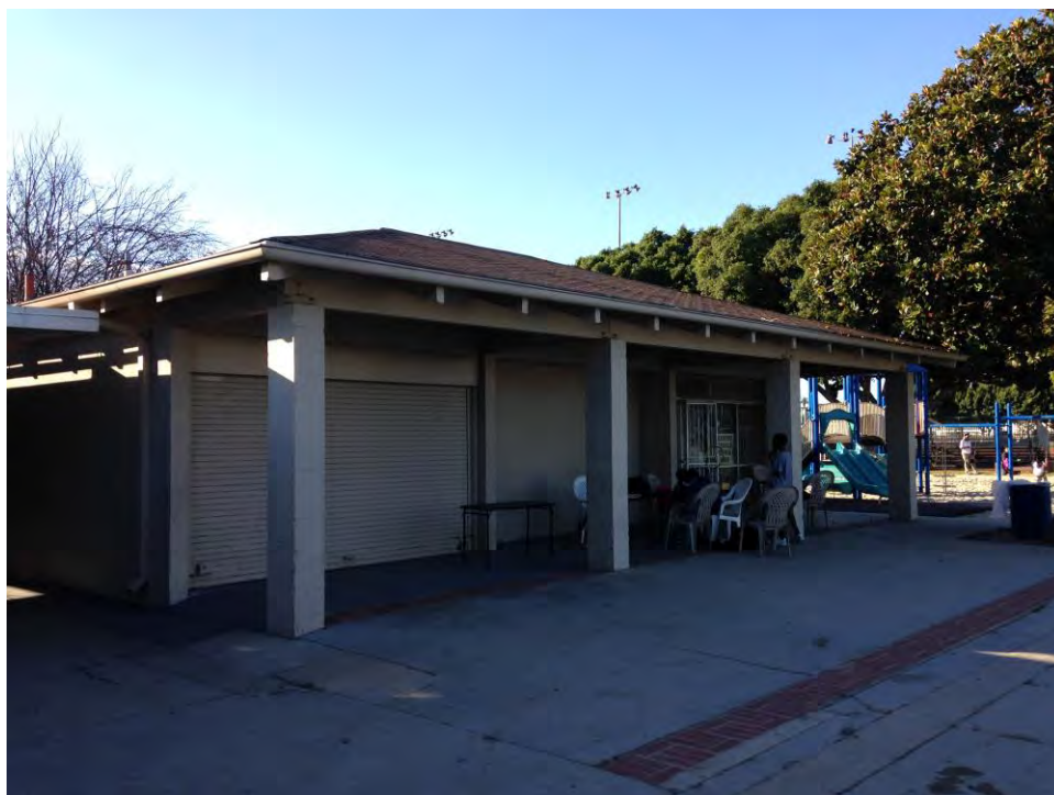
Plate 8. Tennis Shop, view facing northeast
