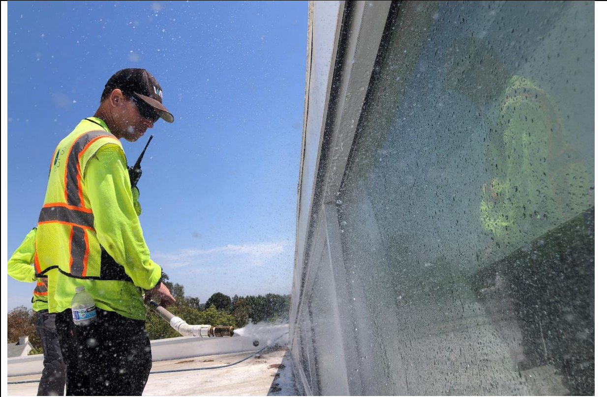
Photo 87: Diagnostic testing was carried out at the two southernmost ribbon windows.
