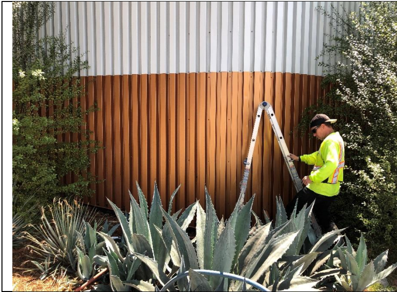
Photo 78: Diagnostic testing preparation on the west side of the building.
