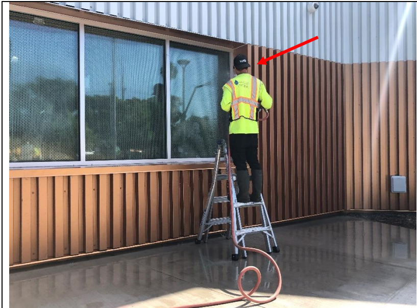
Photo 74: Overview of diagnostic testing on the south side of the building.
