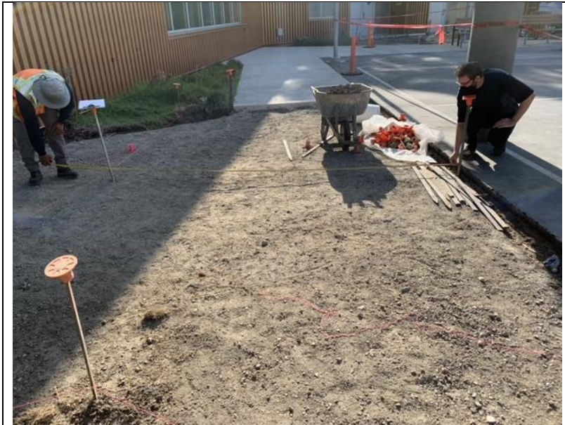
Photo 94: Photo during the replacement of the sidewalk.
