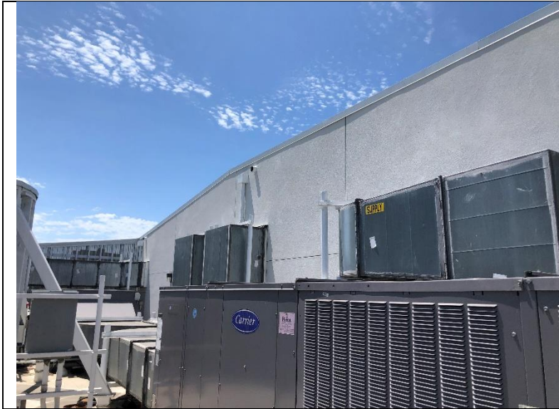
Photo 04: An overview of the lower mechanical roof.
