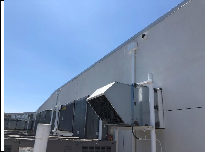
Photo 56: There is not currently a fixed ladder in place to access the upper roof.
