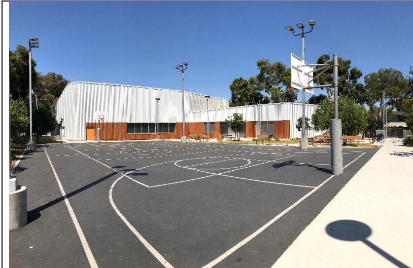
Photo 01: An overview of the south elevation of the recreation center.
