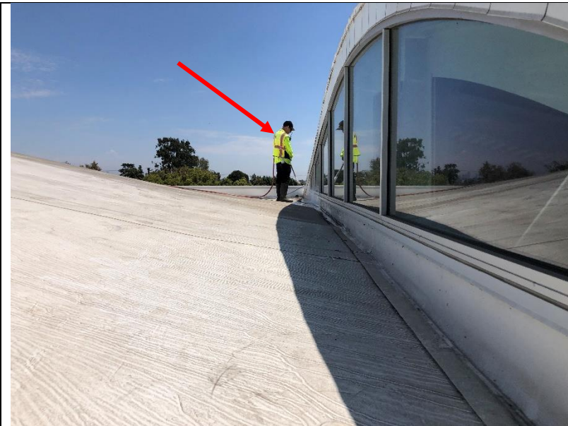
Photo 86: Diagnostic testing was carried out at the two southernmost ribbon windows.
