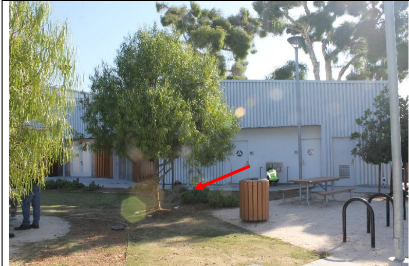
Photo 05: An overview of the south elevation of the recreation center with landscaping at grade.
