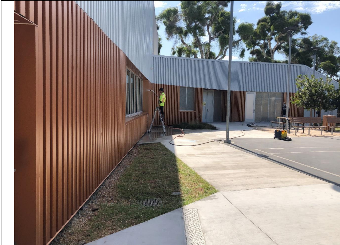
Photo 73: Overview of diagnostic testing on the south side of the building.
