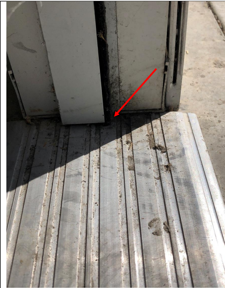
Photo 42: Close-up view of a door threshold.
