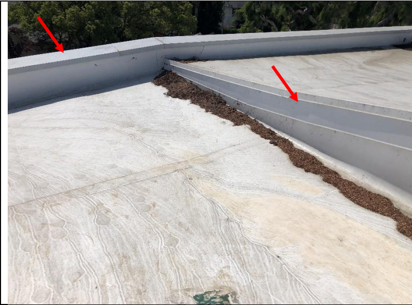
Photo 57: Coping and edge of roof metal on the upper roof.
