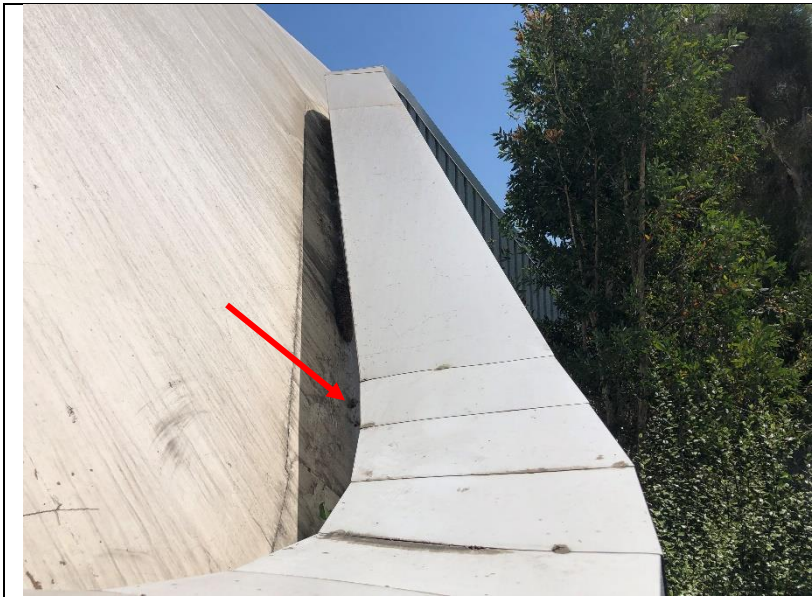
Photo 61: Steep roof slope on the west side of the building.
