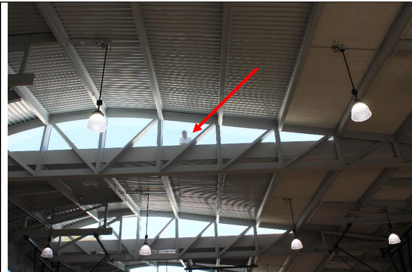
Photo 85: DTR making observations of the ribbon windows.
