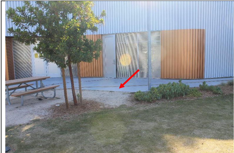
Photo 06: An overview of the south elevation of the recreation center with landscaping at grade.
