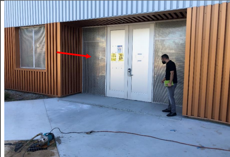
Photo 23: Perforated aluminum panels had been installed at many of the windows.
