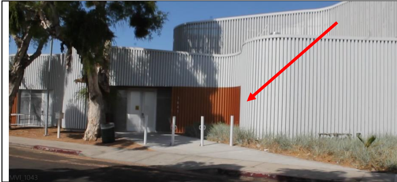
Photo 11: CMU block walls are covered with a corrugated metal cladding system on the east side of the building.
