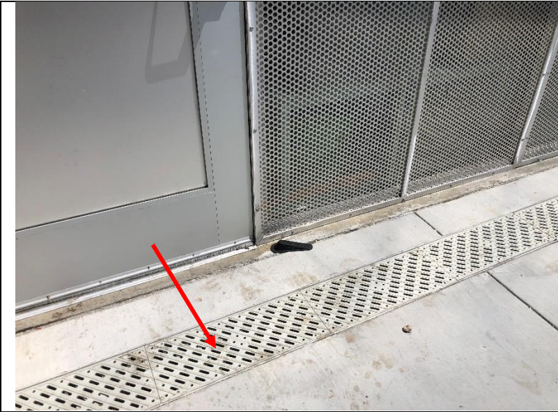
Photo 96: Additional trench drains were installed near doors.
