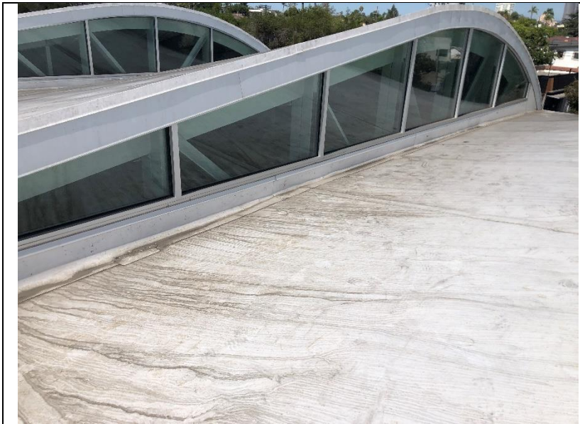
Photo 34: An overview of the vaulted roof over the indoor basketball court.
