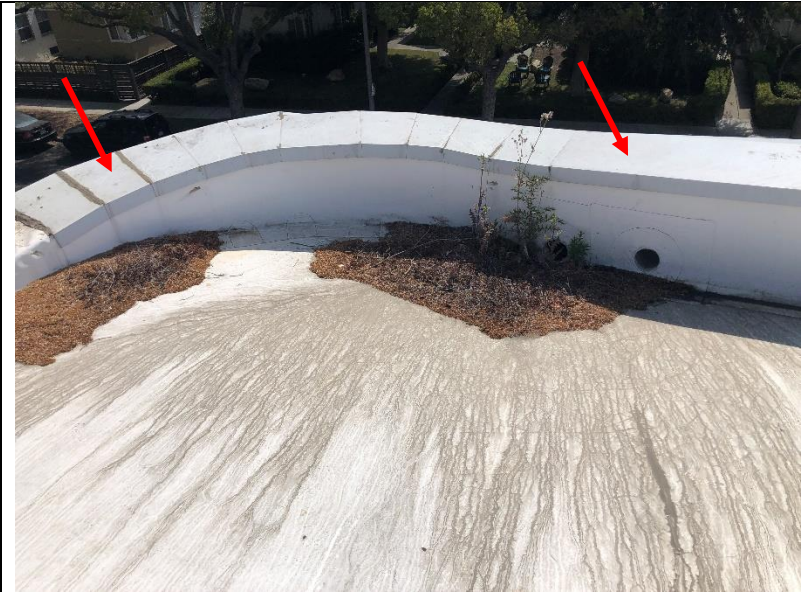
Photo 58: Coping on the upper roof.
