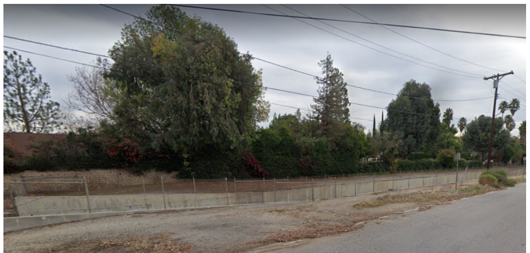
Figure 24: Frontal view of proposed equine trail on Shoup Ave at Valley Circle Blvd
