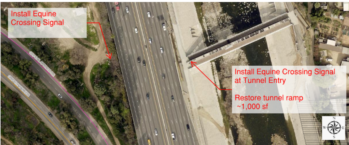
Figure 12: Aerial view of Tunnel One
