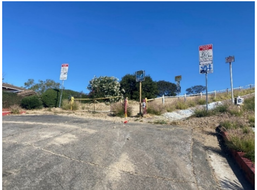
Figure 3: Frontal view of the entrance to Olivia Terrace/Edmore Place Trail
