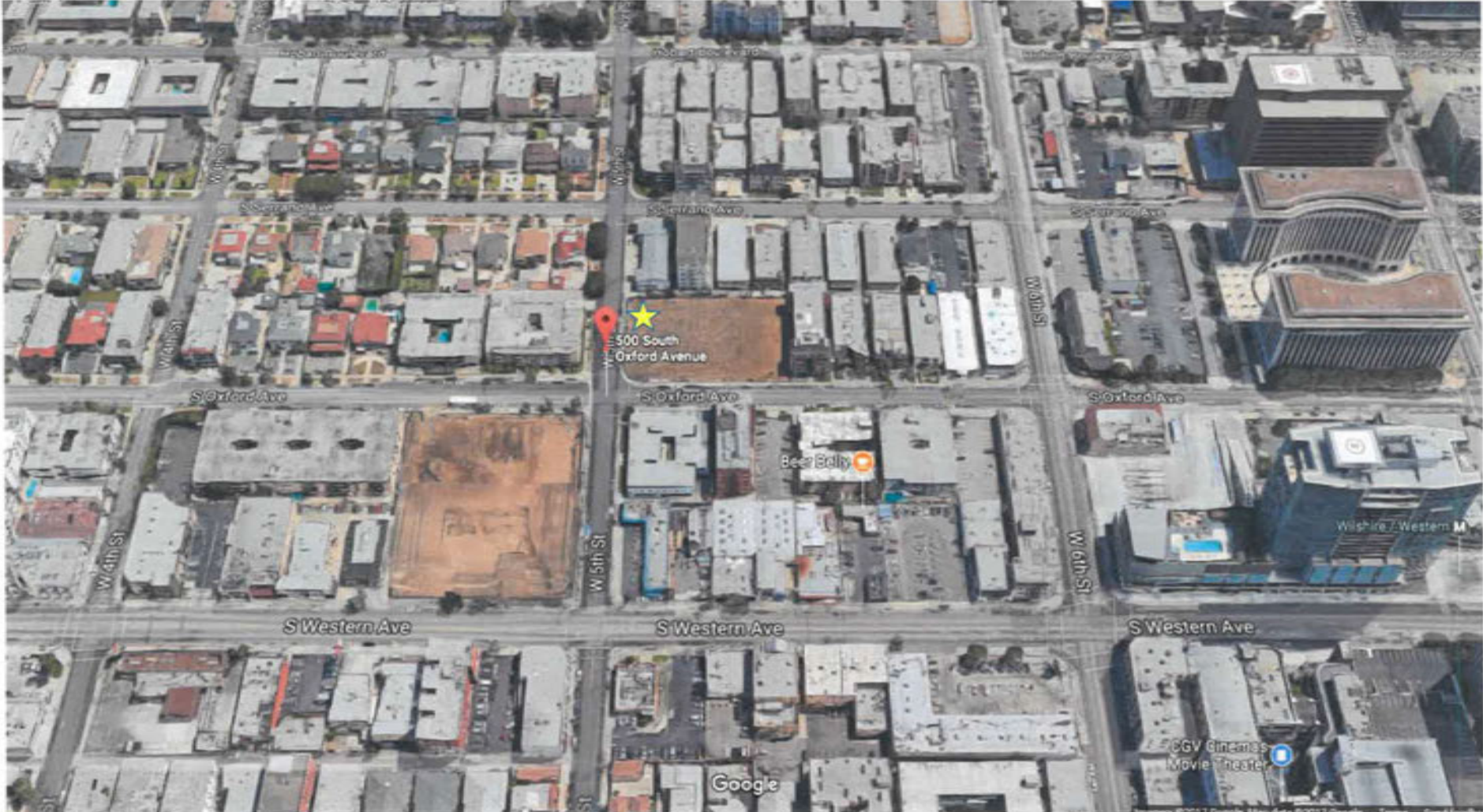
Aerial View of Project Site facing East
