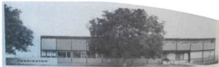
The Torrington Mfg. Co., M. Breuer Architect, 1953
