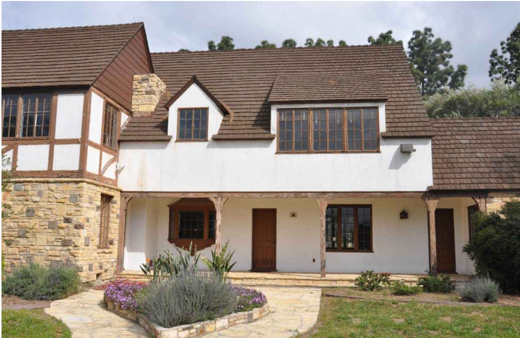
Figure 81: South side of the house and porch, looking north.
