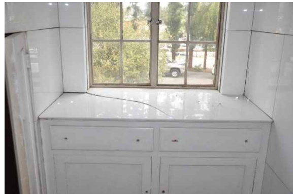
Figure 149: Detail of Vitrolite wall and counter finish.
