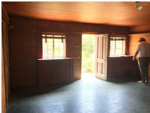
Figure 117: View looking east.
