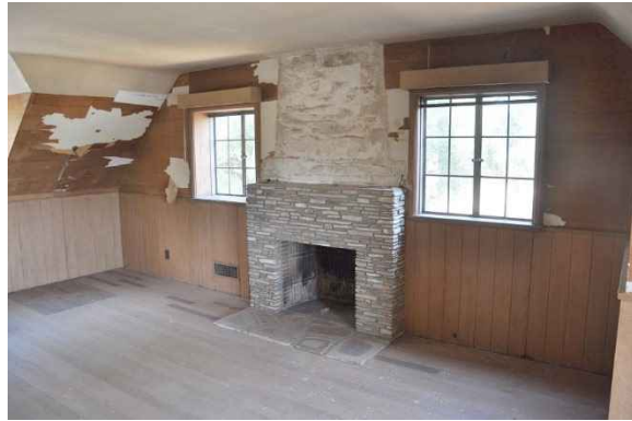
Figure 145: View of the fireplace looking east
