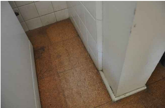
Figure 40: Original cork flooring remains in the kitchen and butler's pantry.
