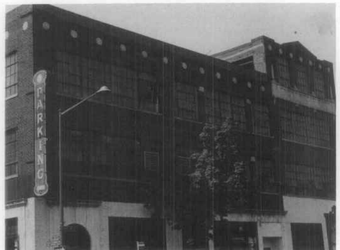
Fig. 5 Windows often provide a strong visual element to relatively simple or unadorned industrial or commercial buildings. This design element should be taken into consideration when evaluating the significance of the windows. Photo: Michael Auer.
