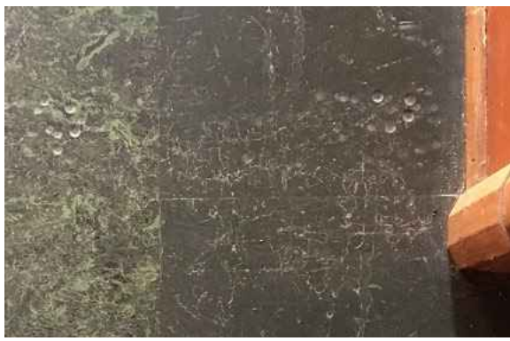
Figure 122: Original flooring remains.
