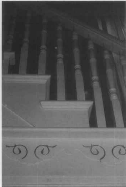
Figure 23. Stair banisters and railings are considered mouthable surfaces. In this case, the old paint was wet sanded to a sound layer. Special encapsulant paints were then applied in three thin layers to avoid obscuring the woodwork's fine detailing. It should be noted that many encapsulant paints are now treated with a bitter agent to discourage mouth contact. Photo: Landmarks Design Associates.
