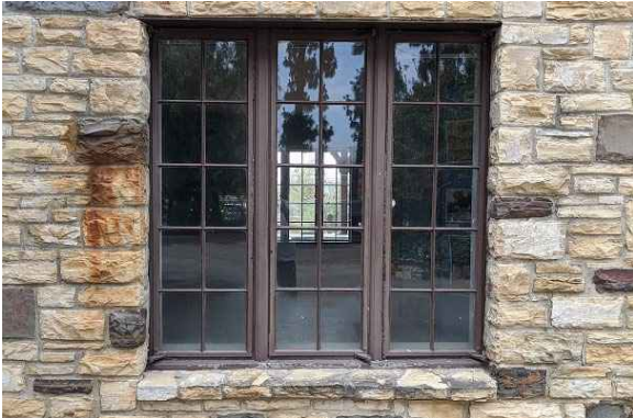
Figure 21: Typical steel window.
