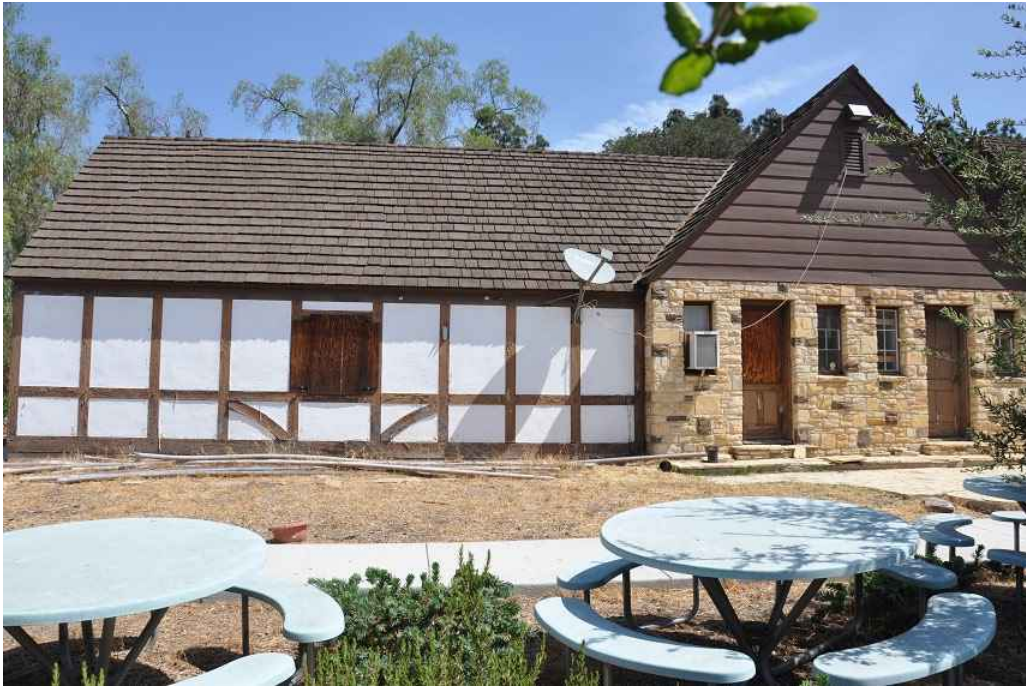
Figure 79: South side of the garage and pool restrooms, looking north.
