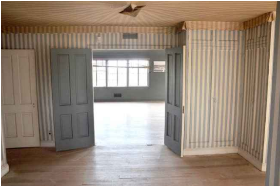
Figure 138: View looking south.
