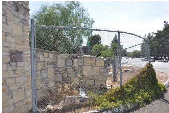
Figure 74: View of the entry gate wall looking northwest.
