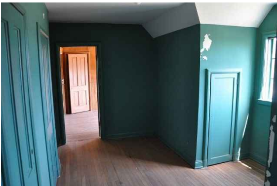
Figure 129: View looking east.
