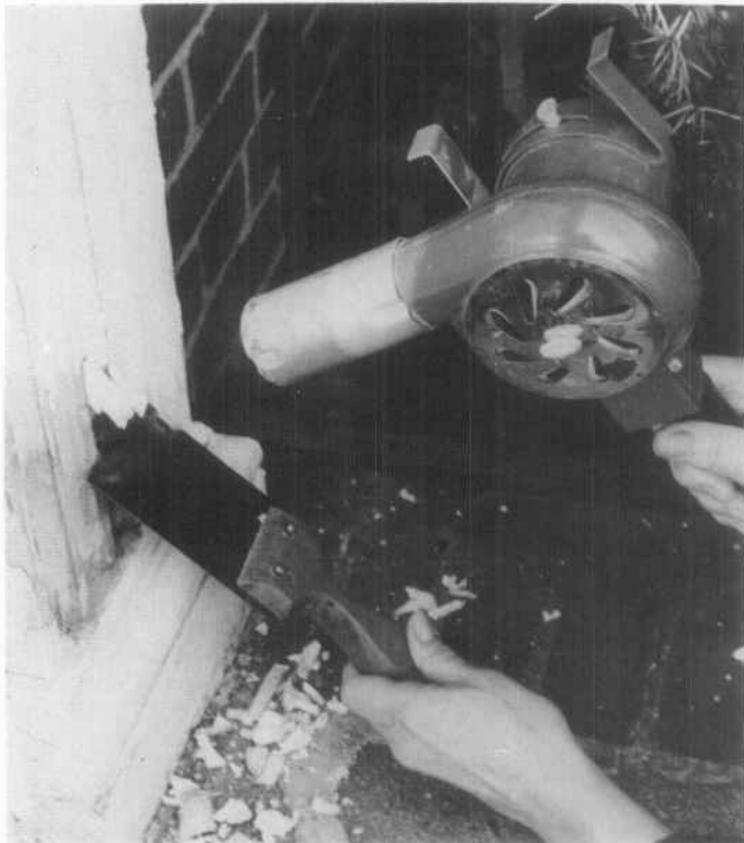
Fig. 14 The nozzle on the electric heat gun permits hot air to be aimed into cavities on solid decorative elements such as this applied column. After the paint has been sufficiently softened, it can be removed with a profiled scraper. Photo: Charles E. Fisher, III.
