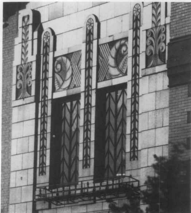
Fig. 1 Often highly distinctive in design and craftsmanship, rolled steel windows play an important role in defining the architectural character of many later nineteenth and early twentieth century buildings. Art Deco, Art Moderne, the International Style, and Post World War II Modernism depended on the slim profiles and streamlined appearance of metal windows for much of their impact. Photo: William G. Johnson.
