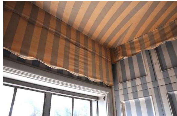
Figure 141: Detail of fabric ceiling finish.
