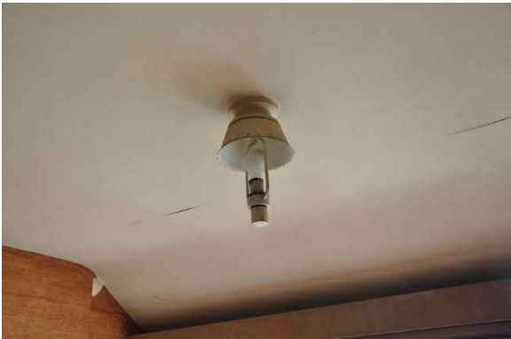
Figure 146: An original light fixture remains.
