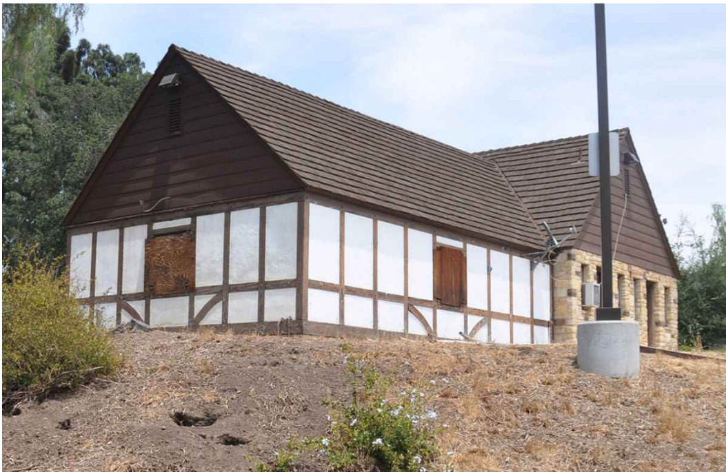
Figure 78: Southwest side of the garage, looking northeast.
