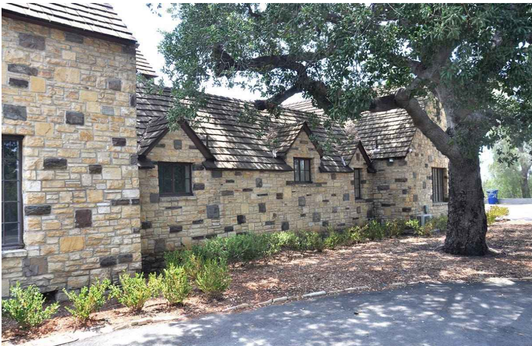
Figure 76: North side of the house, looking southwest.
