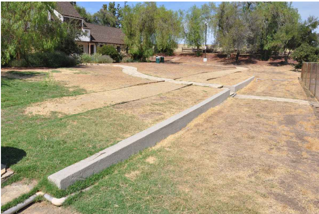
Figure 63: Rear yard zone looking northeast.
