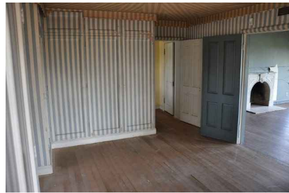
Figure 139: View looking east.
