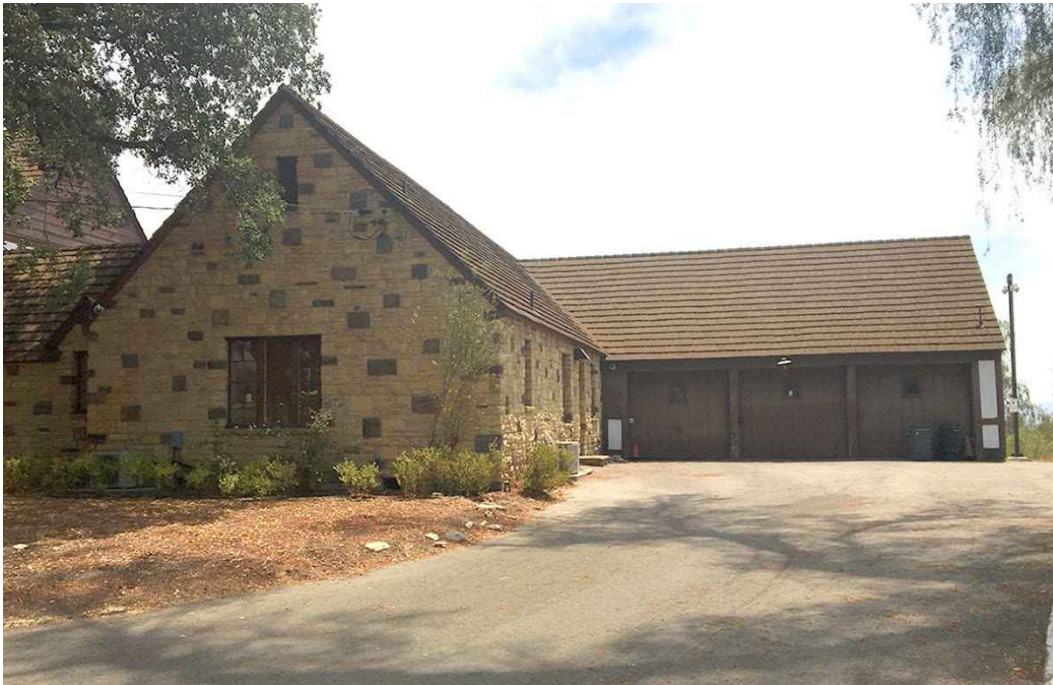
Figure 77: North side of the house and garage, looking south.
