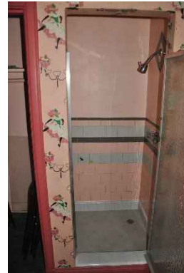
Figure 126: View of shower in "setters" bath.
