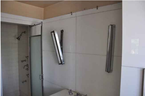
Figure 150: Original wall sconces remain.
