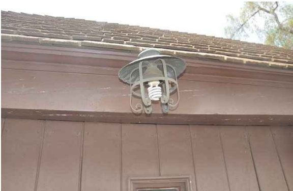
Figure 30: Original light fixture at the garage to be refurbished.
