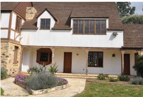
Figure 13: South facing porch looking north.
