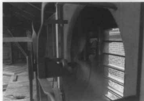
D. Install ventilating fans when additional air circulation will improve damp conditions in buildings or reduce cooling loads. Photo: Ernest A. Conrad, P. E.
