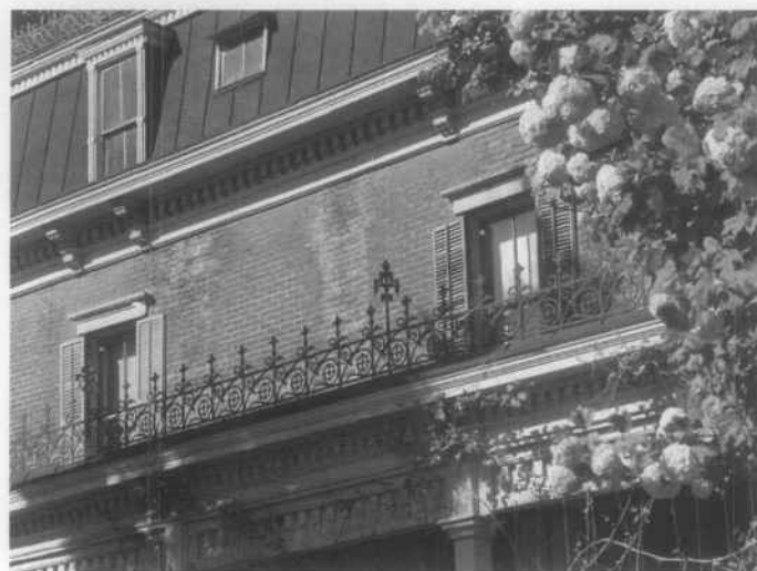
Fig. 4. Deferred maintenance often leads to blocked gutters and downspouts. This cracked gutter system allowed moisture to penetrate the upper exterior wall, erode mortar joints, and rot fascia boards. Photo: NPS files.
