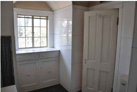
Figure 148: View looking north.
