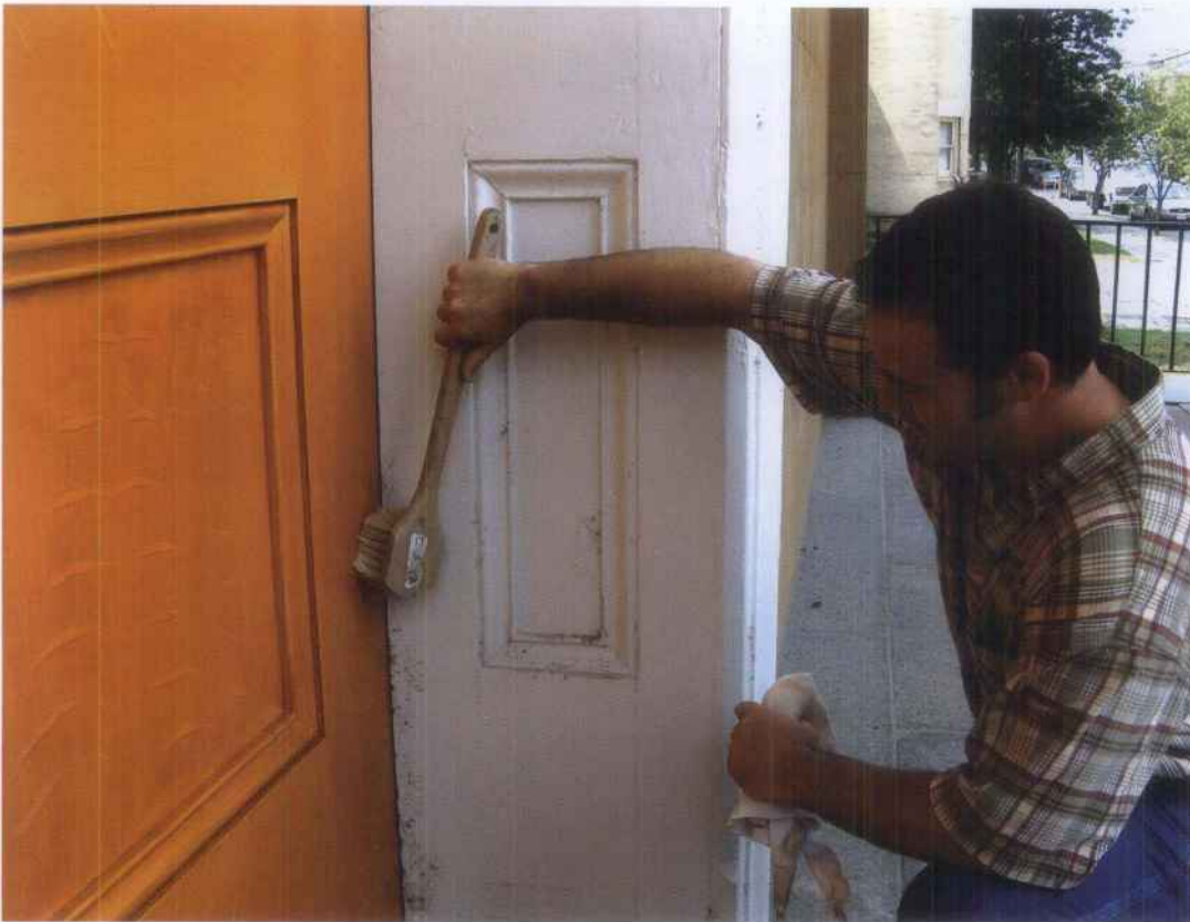
Figure 9. To help extend a repainting cycle, dirt and spider webs should be removed before permanent staining occurs. In this case, a natural bristle brush and a soft damp cloth are being used to remove insect debris and refresh the surface appearance.
