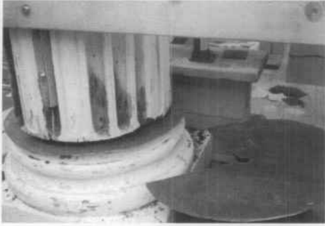
A. This lead sheet was installed at the base of the replacement column to stop rising damp. Photo: Bryan Blundell.
