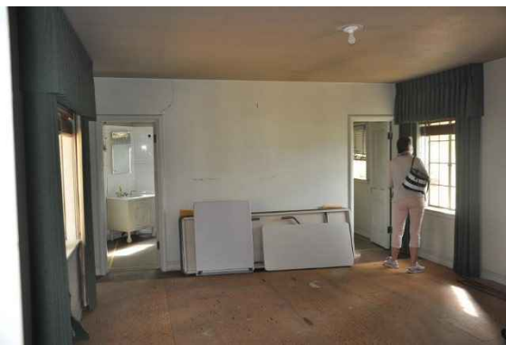
Figure 109: View looking east.
