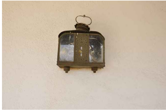
Figure 31: Original light fixture at the south porch to be refurbished.
