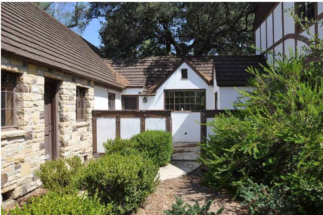
Figure 80: South side of the house and drying yard, looking north.
