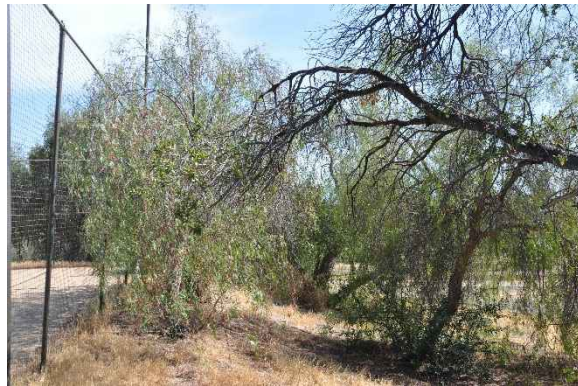
Figure 72: Overgrown vegetation adjacent to the tennis courts. Regular tree and brush trimming will mitigate fire risk and provide more hospitable surroundings.
