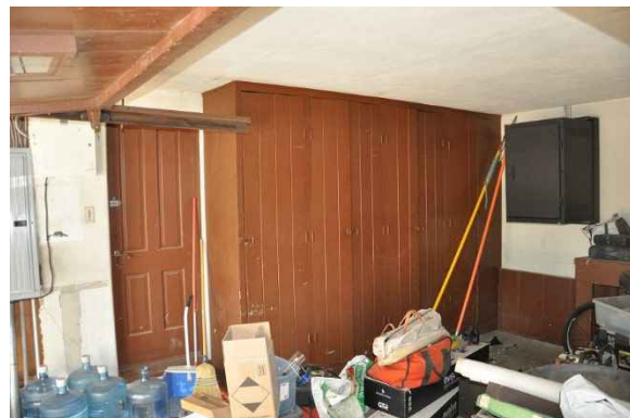
Figure 128: View looking east showing the original chauffer's cabinets.
