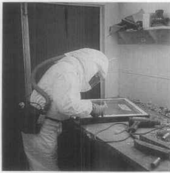
Low-level heat guns can be used to remove lead-based paint from significant historic windows and trimwork, but a worker exposed to lead dust over an extended period of time must be protected from the hazards created during the process of paint removal. Photo: Williamsport Preservation Training Center.
