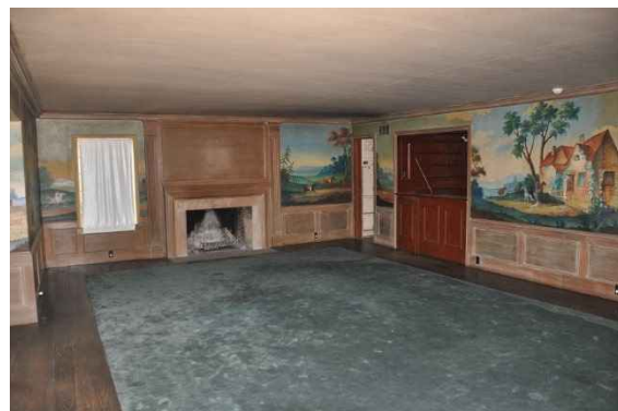
Figure 101: Current condition of the Great Room from a similar angle.
