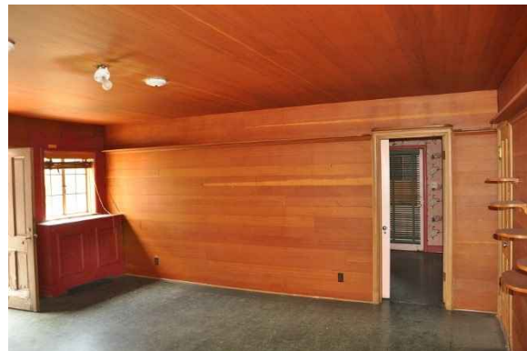
Figure 118: View looking south.
