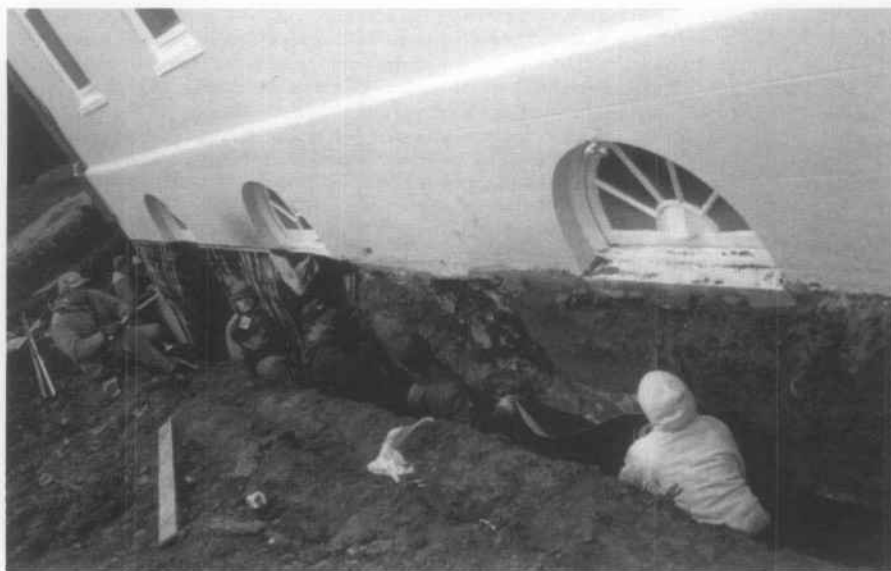
I. Critically damp foundation walls were protected with a layer of bentonite clay to reduce moisture penetration. This work was in combination with new downspouts that were connected to drainage boots that deposited captures roof run-off away from the foundation. Photo: Courtesy, Larry D. Dermody and the National Trust for Historic Preservation.
