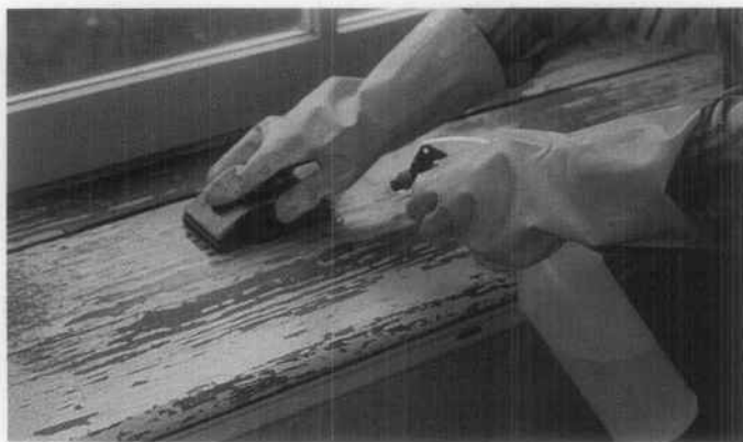
Figure 15. Wet sanding of interior surfaces will keep dust levels down, reduce the need for workers' protection, and provide a sound surface for repainting. Priming and repainting with oil/alkyd, latex or latex acrylic should be undertaken according to manufacturers' instructions.
