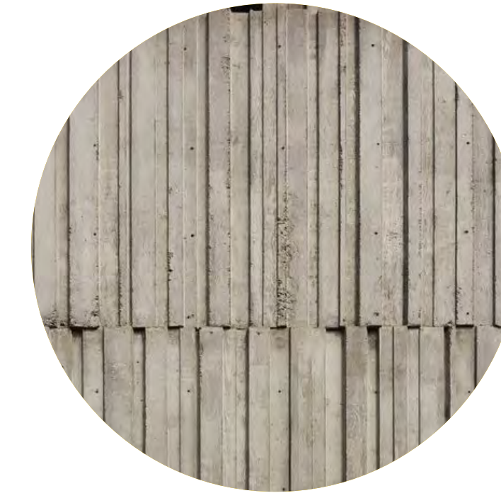
PRECAST CONCRETE WALL
