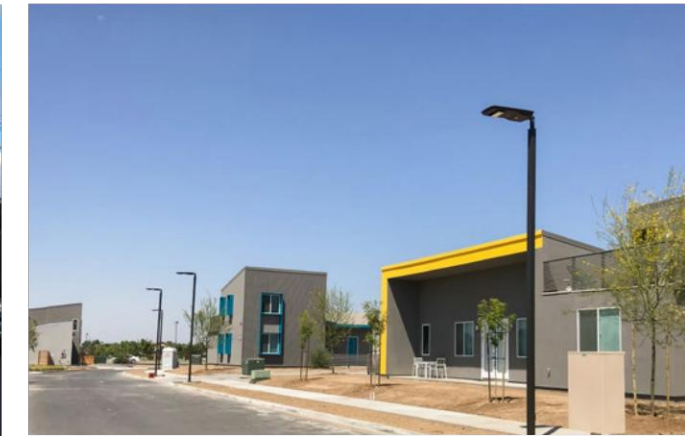
Wonderful Solar Company Delano CA, USA Road Lighting Project
