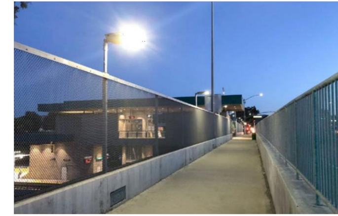
Pittsburg Bart Station Pittsburg CA, USA Pathway Security Lighting Project
