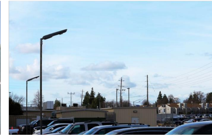
VA Medical Center Sacramento CA, USA Parking Lots Lighting Project
