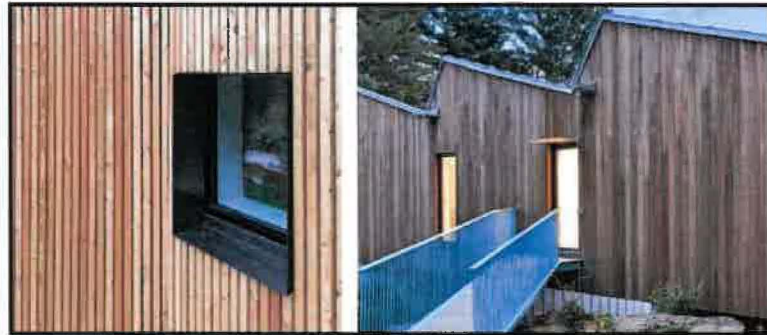
VERTICAL SIDING/PUNCHED RECESSED WINDOWS/VARIED ROOFLINES
