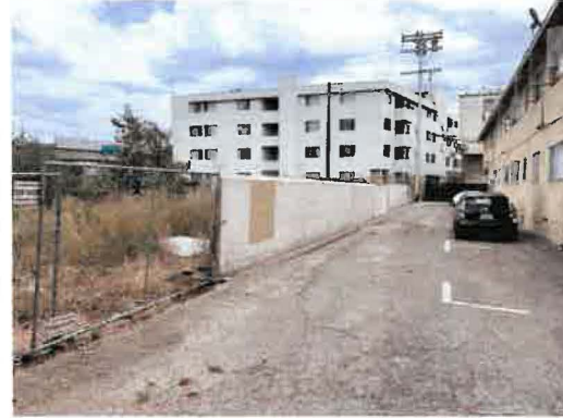
SOUTHERN PROPERTY WALL BETWEEN SITE AND NEIGHBORING 2-STORY MULTI-FAMILY BUILDING
