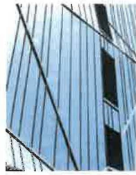
STANDING SEAM ZINC METAL PANEL STAGGERED PATTERN - PIGMENTO BLUE
