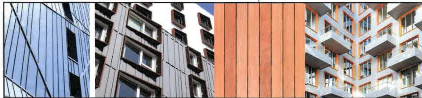
STAGGERED STANDING SEAM SIDING/RECESSED PUNCH WINDOWS/SUNSHADES/VERTICAL SIDING/ACCENT
