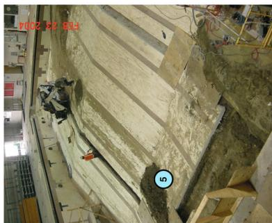
PROBLEM: DETERIORATED & CRACKED SUPPLY WATER UNDER POOL OR RETURN LINES LEAK WATER.
