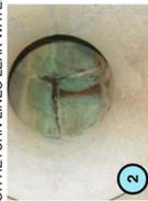
PROBLEM: CRACKS IN SUPPLY OR RETURN WATER SYSTEM UNDERMINES POOL BOTTOM AND CREATES CRACKS.
