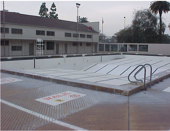
Lincoln Park Pool—the #1 replacement priority for the Department city-wide
