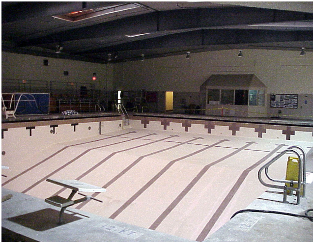
A refurbished E.G. Roberts will reopen later in the summer of 2004
