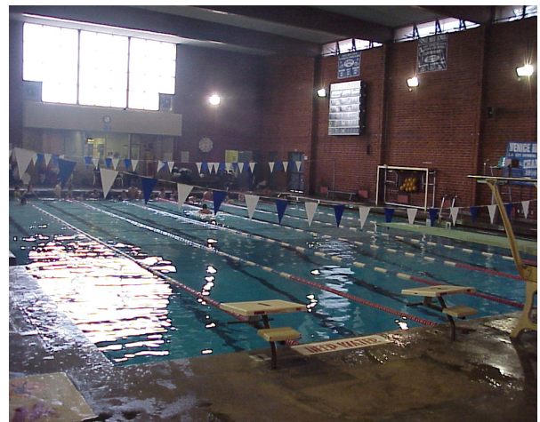
Leaking pipes at Venice make keeping the pool open a daily challenge.
