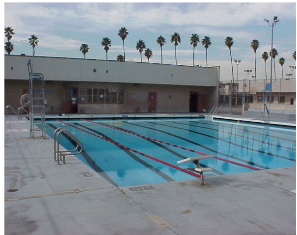
Banning needs major bathhouse work.
