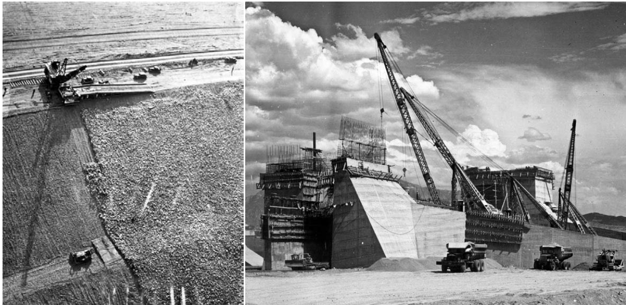
Construction of the Dam
