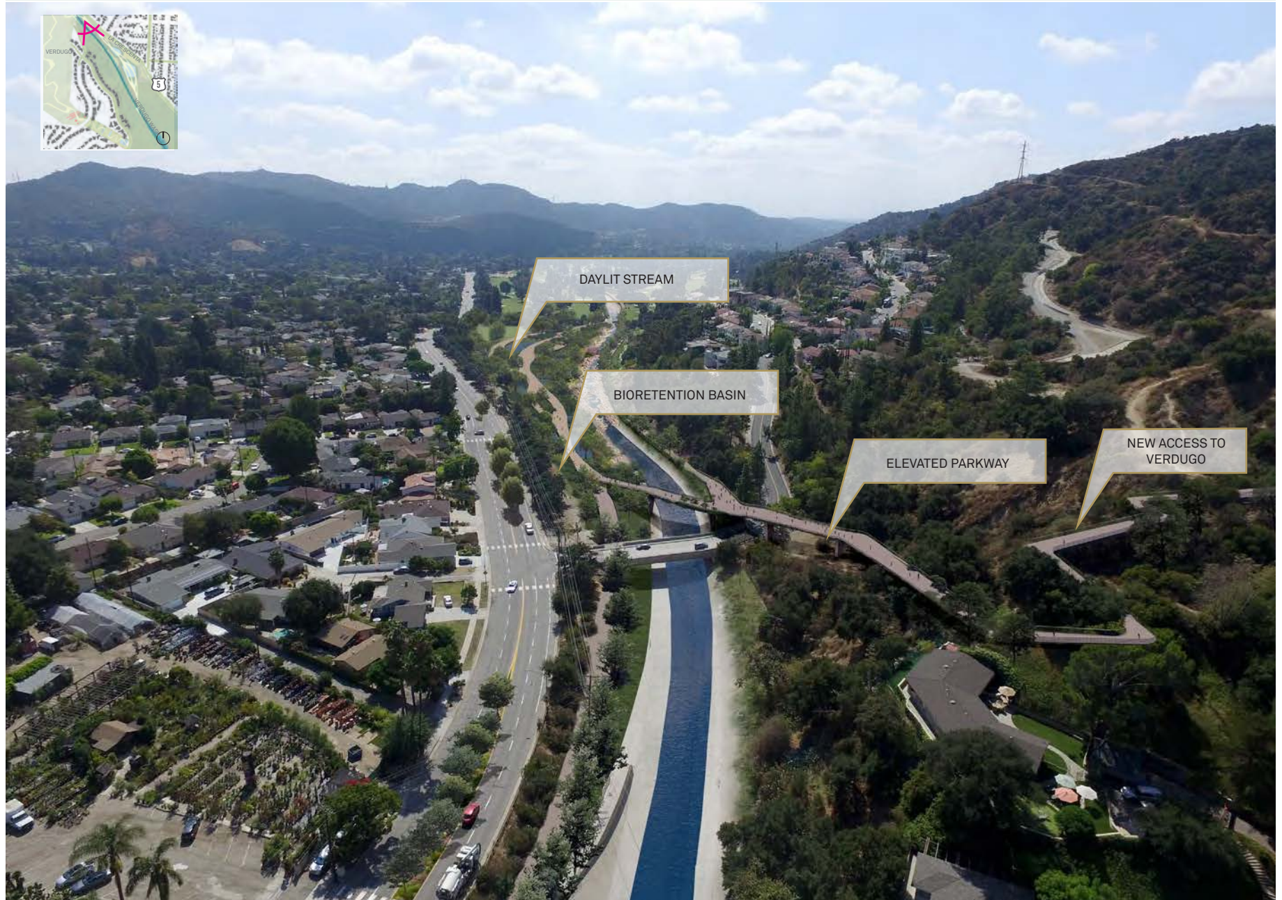
View looking South at Verdugo Wash and Invale Drive
