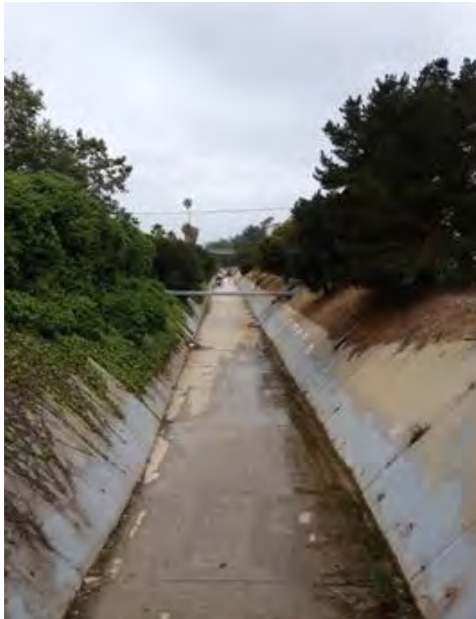
Original Configuration of Caltrans Channel
