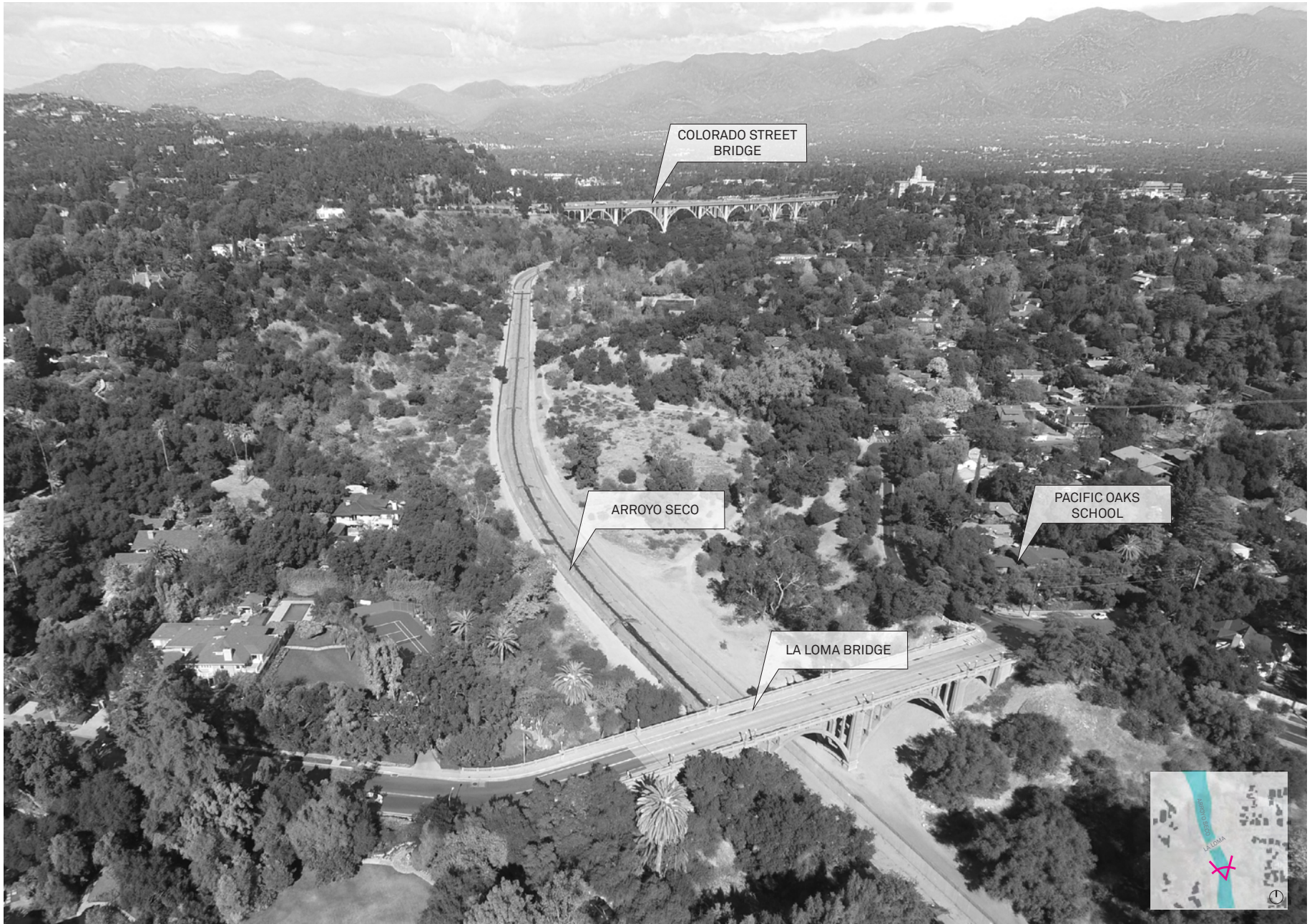
Existing Conditions looking North from Bradford Street
