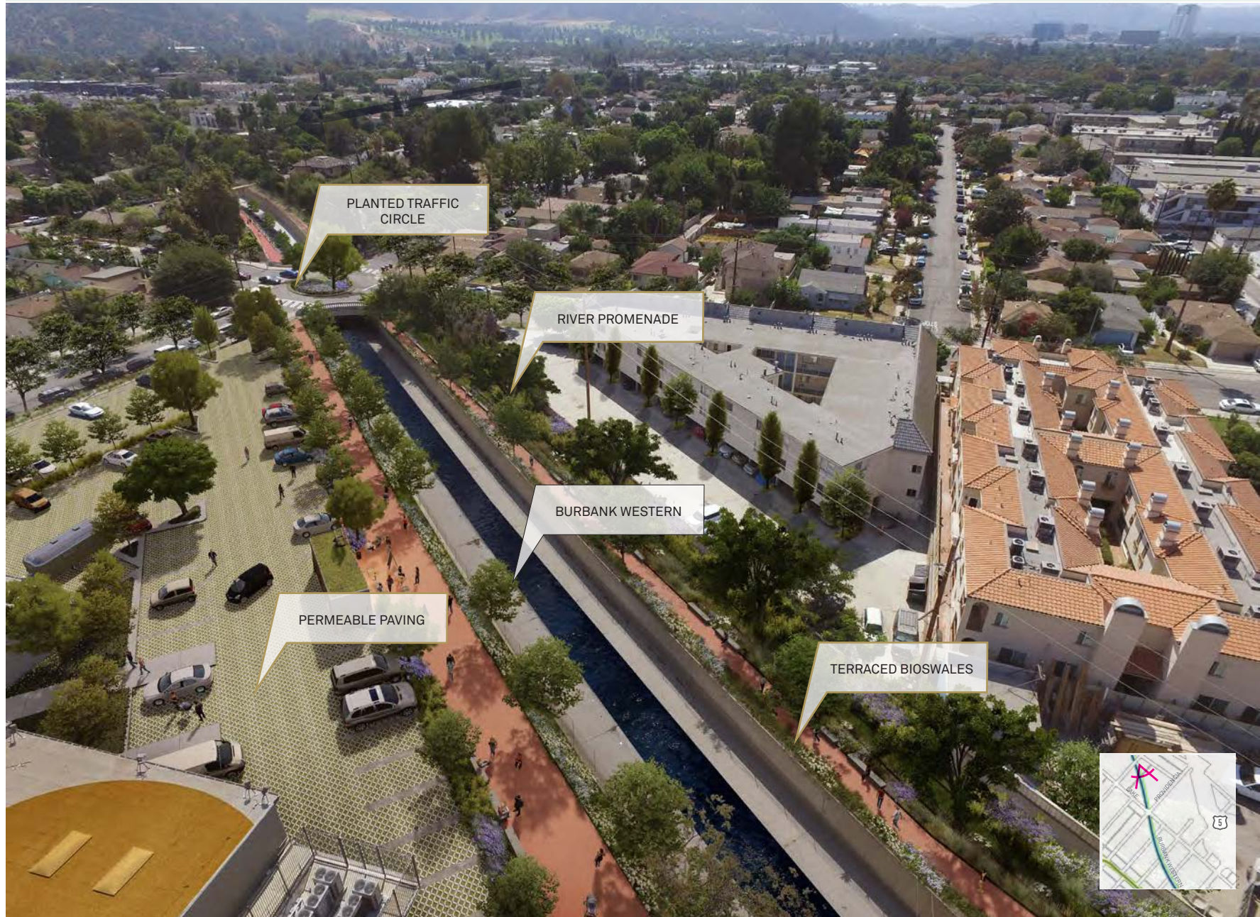
View looking South at Burbank Western Channel and South Lake Street
