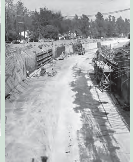
1949: Construction of channel walls for Valley Flood Control Plan
