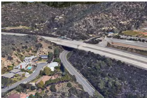
Existing Tunnel under the CA-2
