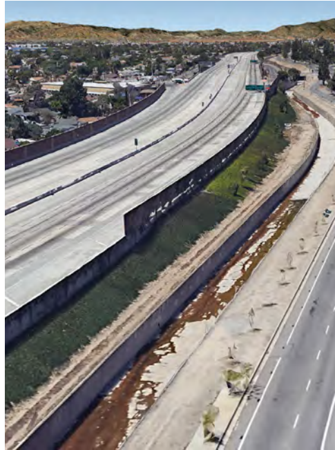
Burbank Western Channel (in this area)
