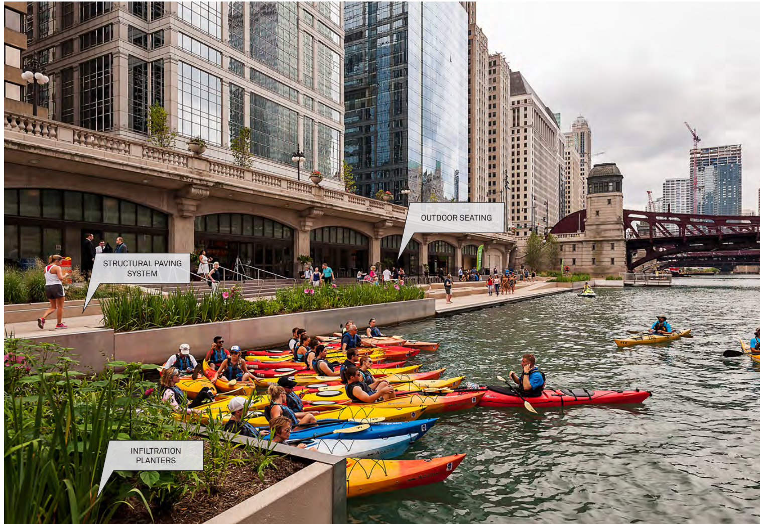
Chicago Riverwalk (Chicago, IL) offers a connected and well-proportioned series of commercial spaces on the south bank of the Chicago River’s main branch. The design includes a buffer zone between the development and the river with infiltration planters and a structural paving system that enables soil volumes and irrigation using reclaimed stormwater.
