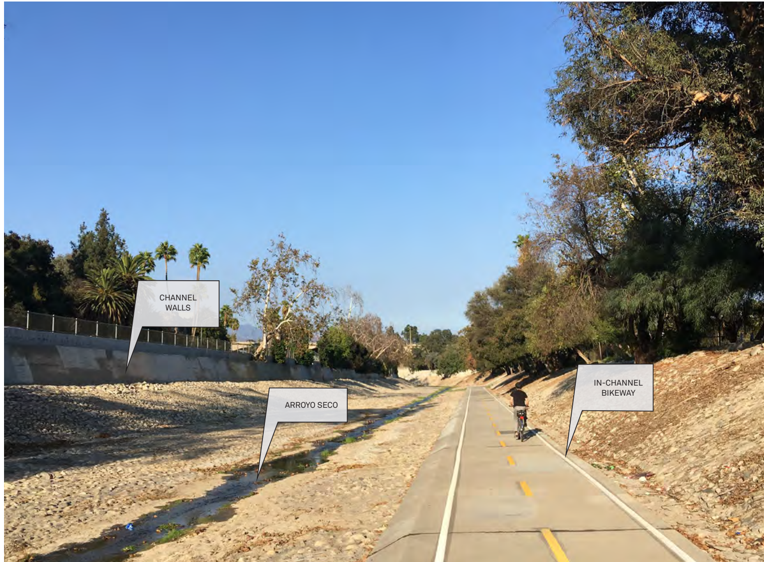
The Arroyo Seco In-Channel Bike Path (Pasadena, CA). A continuous path along the waterway provides grade-separated connection along the bottom of the channel. In-channel bike paths provide a lower cost alternative to bridge modifications and re-building efforts.
