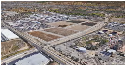
Hansen Spreading Grounds
