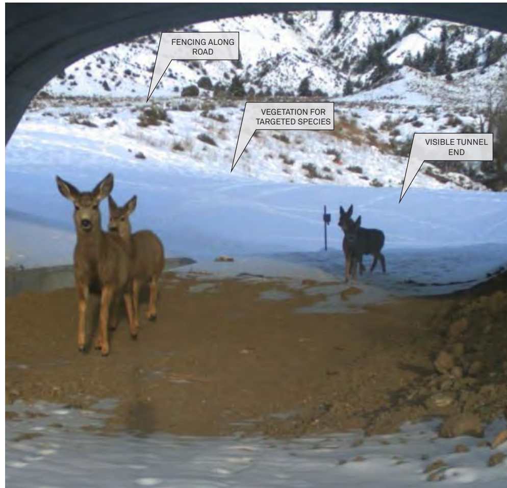
Colorado State Highway 9 Wildlife Underpass (State Highway 9 between Green Mountain Reservoir and Kremmling, Colorado) showcases some key criteria for wildlife crossing that were mentioned in the Caltrans Wildlife Crossing Guidance Manual. First, it is wide enough to allow mammals to see habitat and light on the opposite side of the culvert (Wildlife may perceive danger in underpasses that are too narrow). This underpass also works in conjunction with highway fencing and vegetation to help funnel wildlife toward the corridor.
