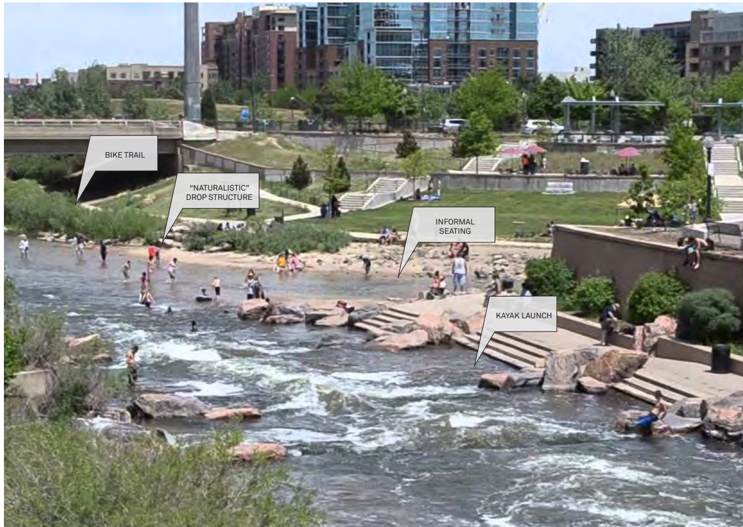
Cherry Creek (Denver, CO). For 40 years, Cherry Creek was a single-purpose channelized flood-control infrastructure device. Starting in 1996, a urban renewal plan modified the creek and revitalized creek-front neighborhoods. This included day-lighting portion of the covered stream, removing parts of the concrete walls, and building bike trails along the creek. Naturalistic drop structures were built that provided informal pedestrian areas while simultaneously stabilizing the channel bottom.
