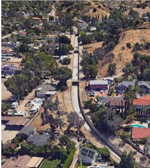
Burbank Western Channel (in this area)
