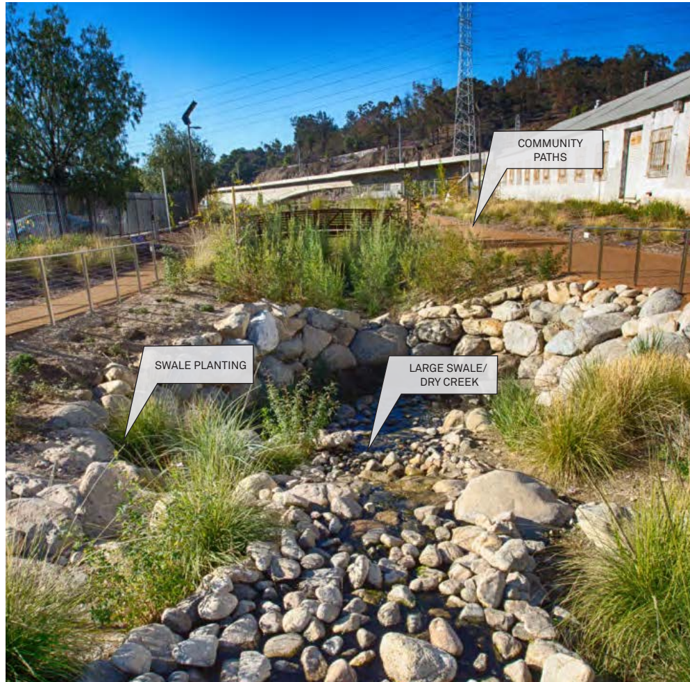
Ed P. Reyes Greenway Stormwater Treatment Swale (Los Angeles, CA). Located on the north bank of the Los Angeles River, this park converted a former street-end into a “stormwater greenway” that cleans water within its 135-acre drainage area. The park feature mimics a dry-creek or arroyo ecosystem that supports biological communities and filters/cleans runoff of bacteria, oils, and other pollutants before it enters the River.
