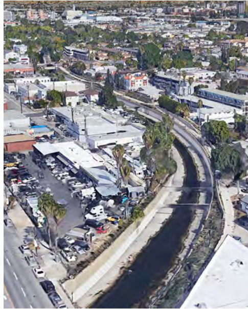
Burbank Western Channel (in this area)
