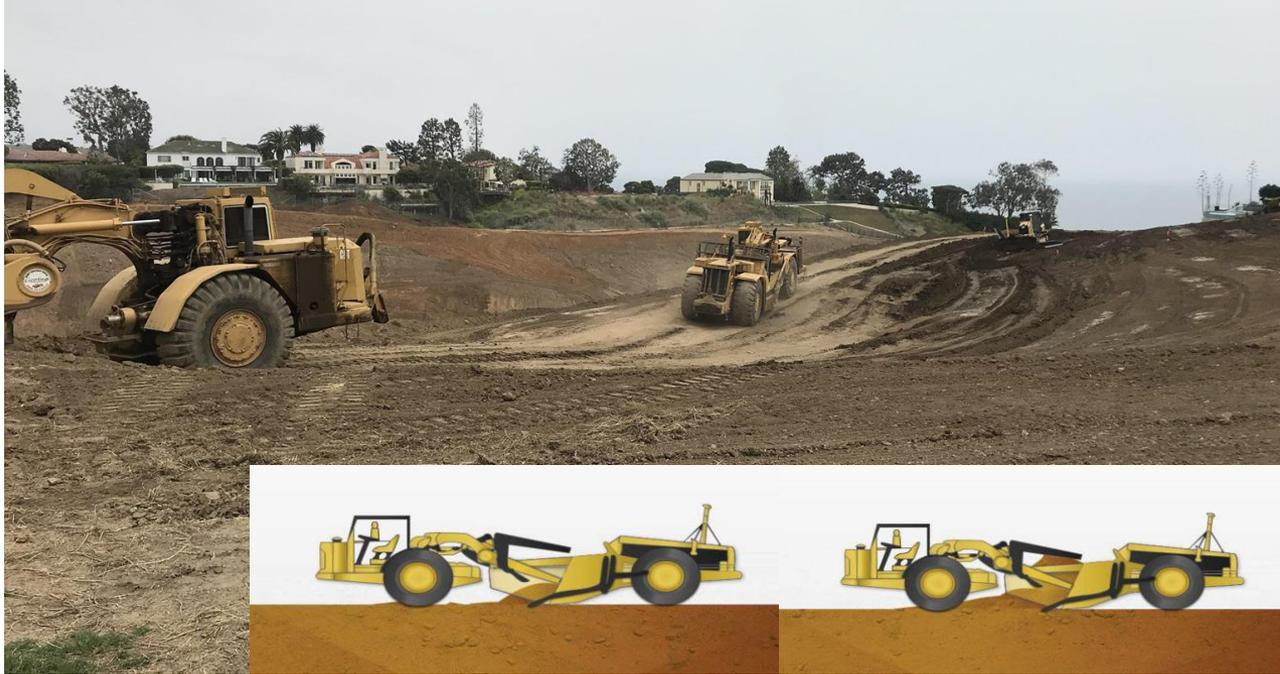
Scrapers are capable of massive grading operations by picking up layers of soil a few inches thick over a long length of haul and so inherently require a large amount of earthwork for access roads and maneuverability. This means that small adjustments in excavation depth may result in relatively large grading areas. With as many as 7 scrapers on the job it is not cost effective to put them on hold while smaller more precise equipment removes the unsuitable soil/debris/mud.
