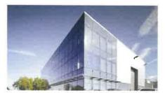
GL-3 \_ Frit Pattern | Garage Facade, Canopies Throughout VE1-2M Clear Insulated Unit; Frit Pattern - 3rd Surface
