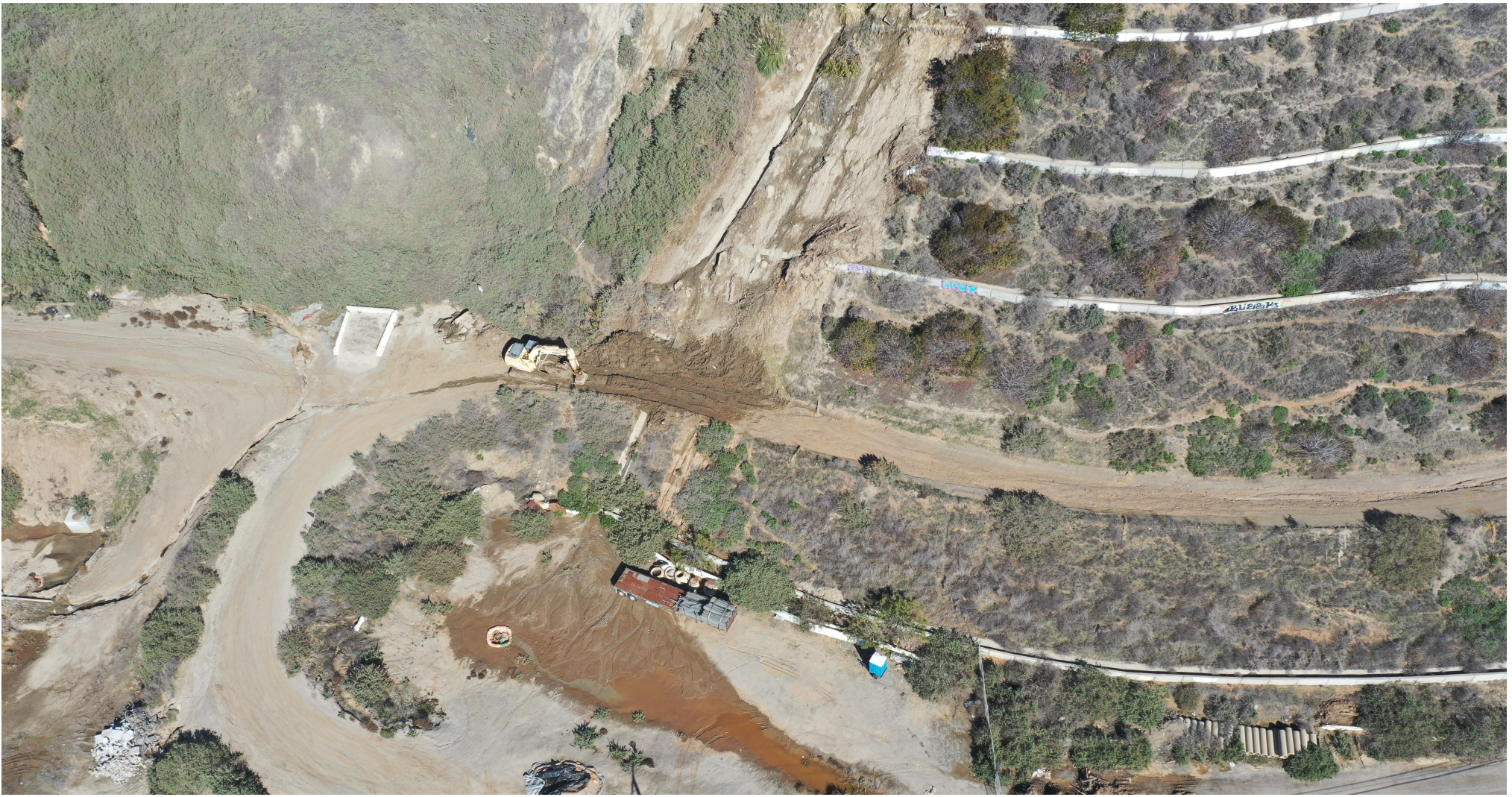
Photo 7: Looking northeast from Pacific Coast Highway. A landslide deposited mud and debris onto the access road. Severe erosional rutting also prevented access to the project stockpile as shown on the left.
