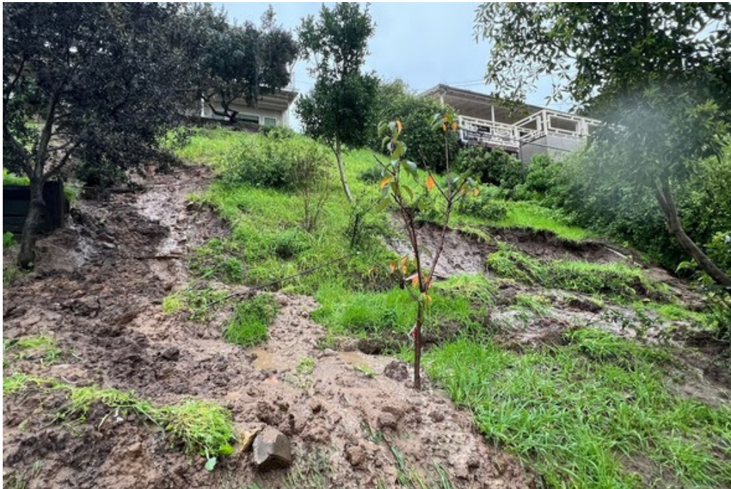
Photo of rainy conditions causing mudflow issues behind homes on Cranks Road.
