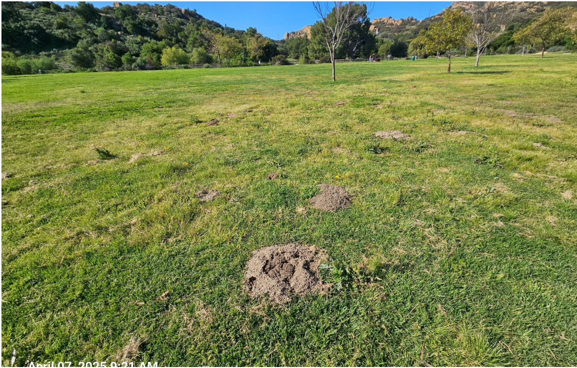
19. Typical burrowing animal hole visible throughout the cap area
