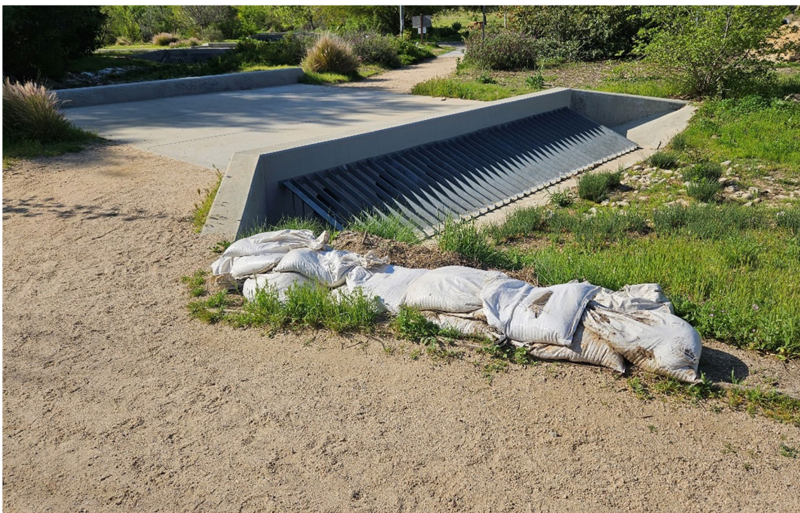
21. Significant swale erosion area near tennis courts showing repair and BMP
