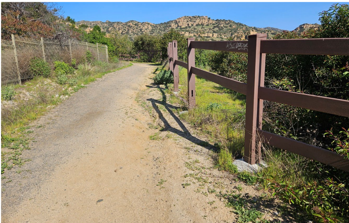
22. Typical shallow erosion repair using degraded granite along pathways
