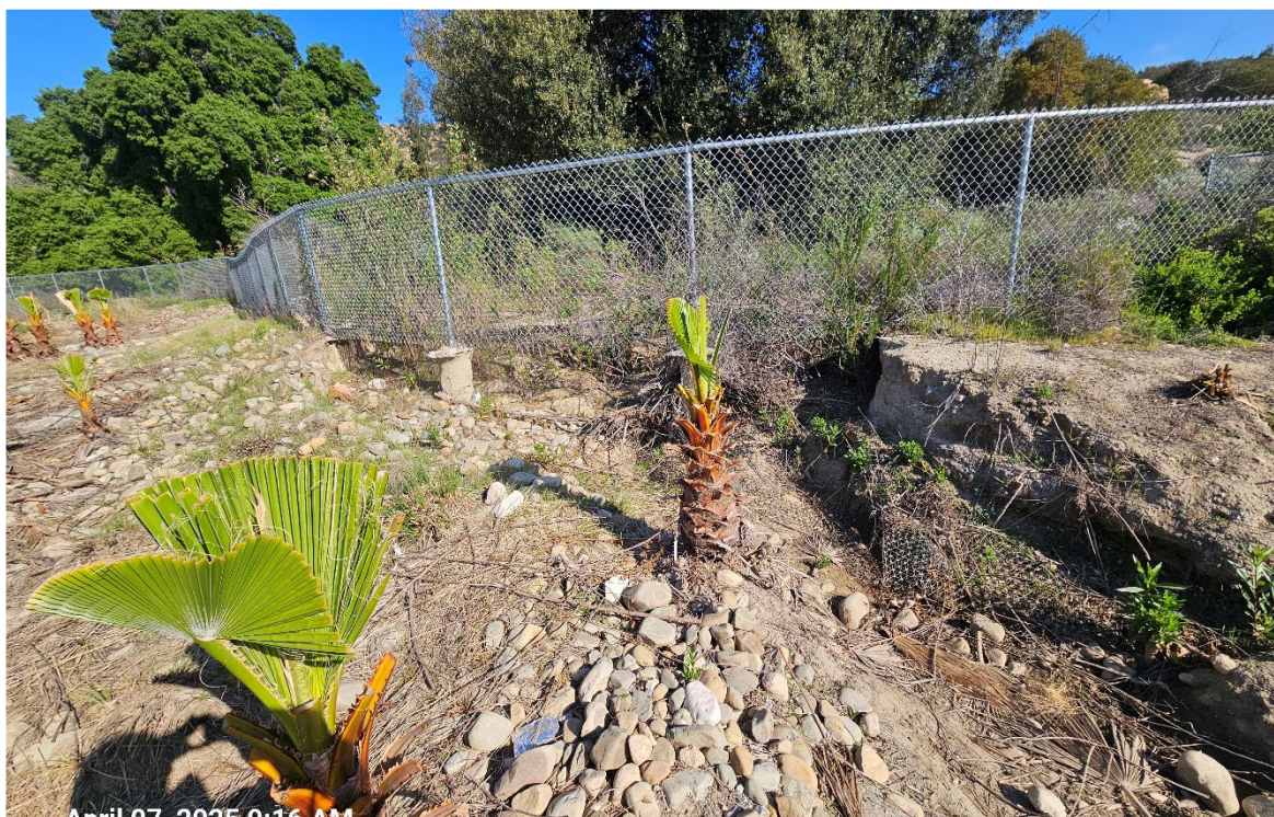
14. View of significant erosion beneath geo grid along swale near northwest end of Site
