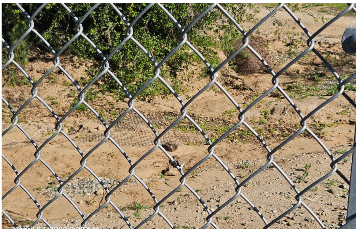
11. View of eroded area behind community center playground with exposed geo grid
