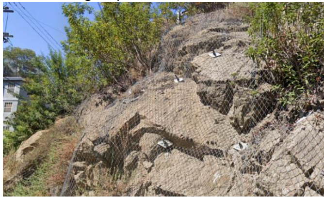
Photo 1: Proposed rock anchored mesh system depiction.
