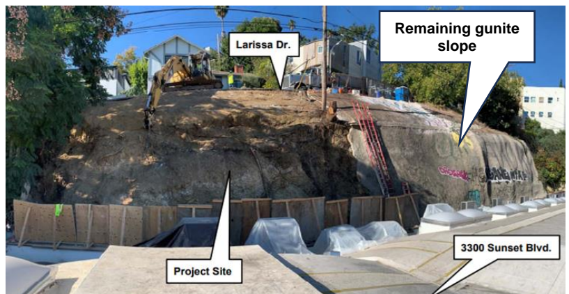
Photo 3: Standing on the roof of 3300 Sunset Boulevard looking west towards the Project site. This photo was taken on December 12, 2023, during demolition and removal of the failed portions of gunite. Note the remaining gunite in the Northern portion of the Project Site
